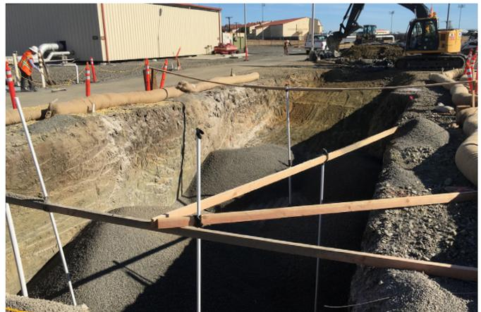
*Travis Air Force Base built the first ever subgrade biogeochemical sulfate reactor that relies on sulfate reduction to biologically treat petroleum contamination in soil and groundwater.*
